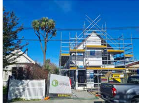
Near complete new Hendon St apartments alongside a traditional villa
